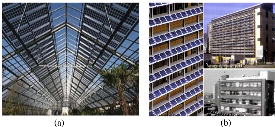
Figure 12: (a) Semi-transparent PV modules integrated into a greenhouse roof; (b) Opaque and semi-transparent PVs used as shading in the Energy Research Centre in Northland (Basnet, 2012).
