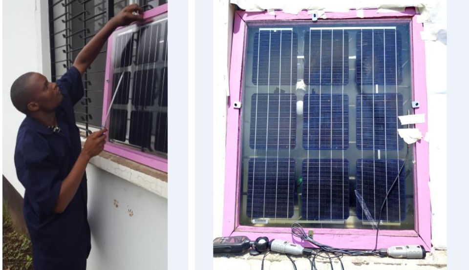
Figure 15: Fixing of the semi-transparent PV and already installed solar panel.
