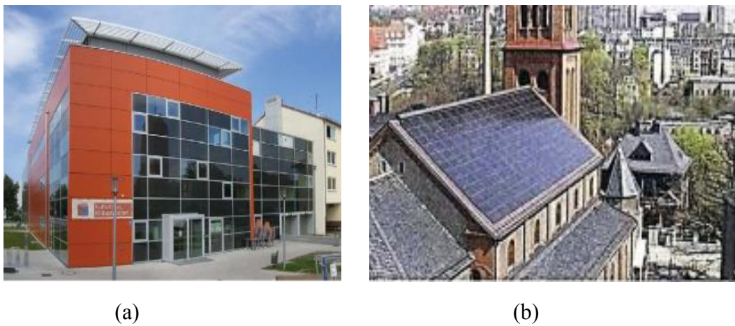
Figure 11: (a) Facade with black micromorph and semi-transparent thin-film modules in Germany and (b) Rooftop application of opaque photovoltaic modules in the Netherlands (Kha, 2013).
