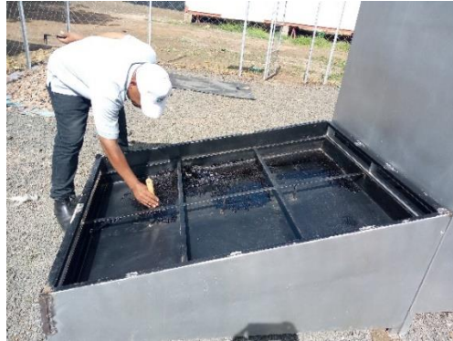
Painting of tarmac/tar in the solar collector
