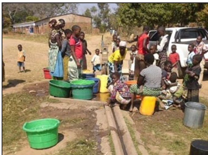
Plate 6.1: A borehole in Thyolo District, Malawi, fitted with an Afridev hand pump
