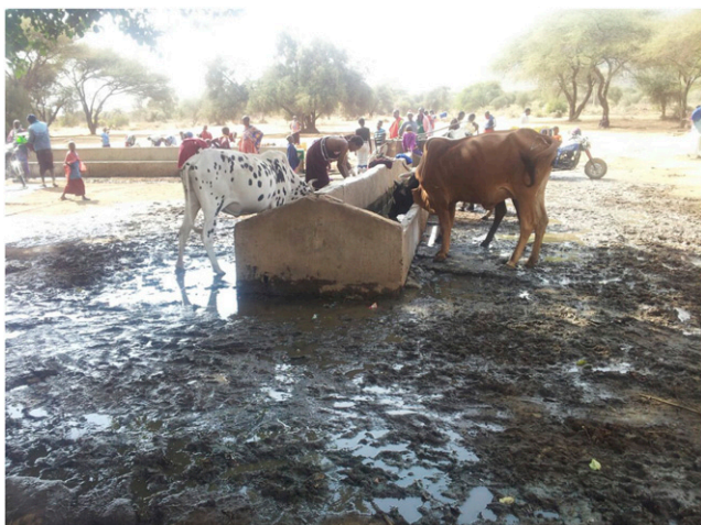
FIGURE 2. Unprotected borehole in Orbomba village at Longido District. This figure appears in color at www.ajtmh.org .
