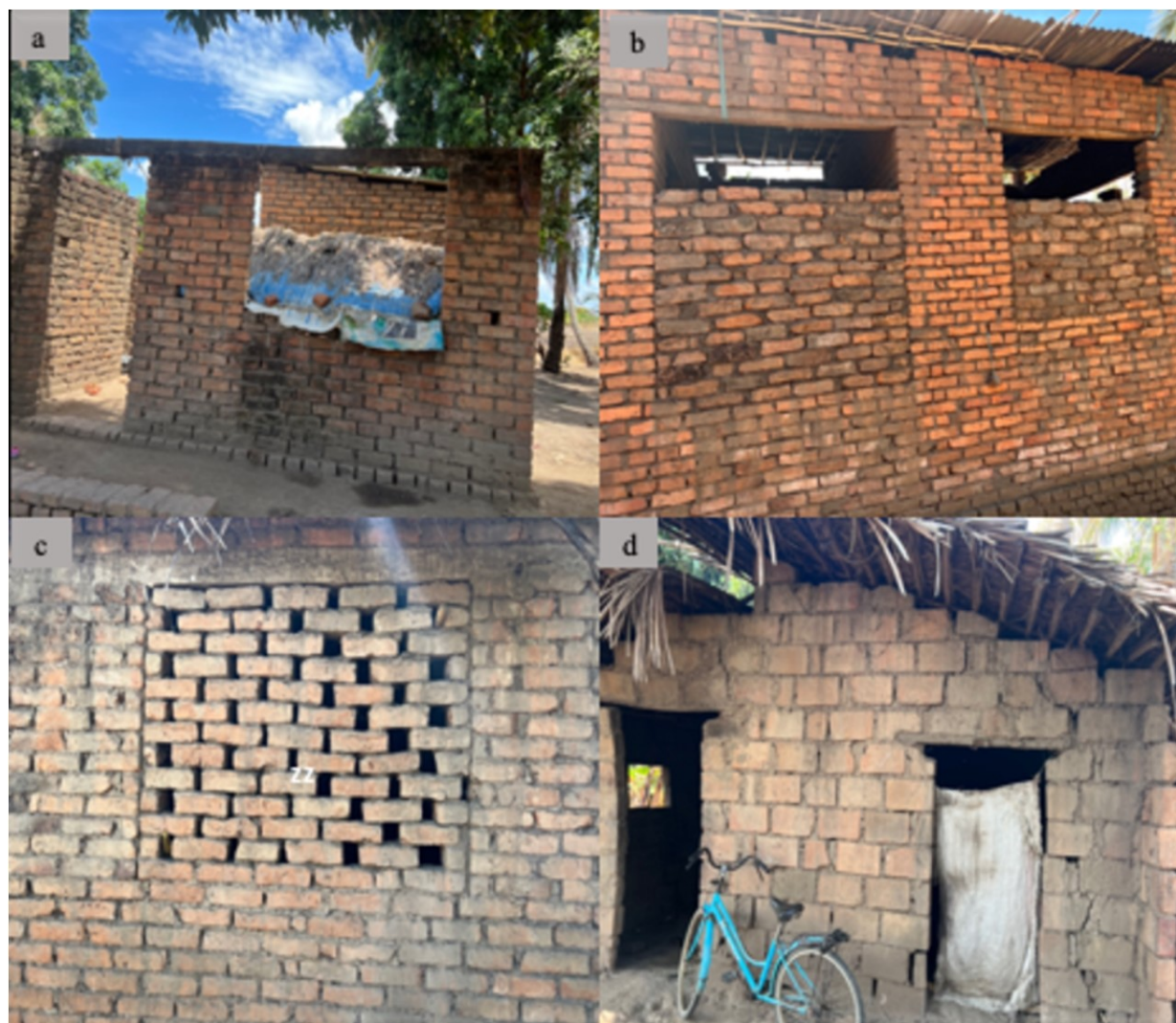
Figure 8: Examples of improved but incomplete houses that people were residing in: (a) un-roofed house, (b) bricks on windows with small gaps on top, (c) holes on the walls and open eaves and (d) no door or window covers installed
