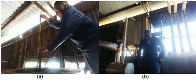
Fig. 1. RABEC Fuel monitoring (a) using a stick and a manual meter (b) descent of the RABEC operator from the top of the fuel tank.
