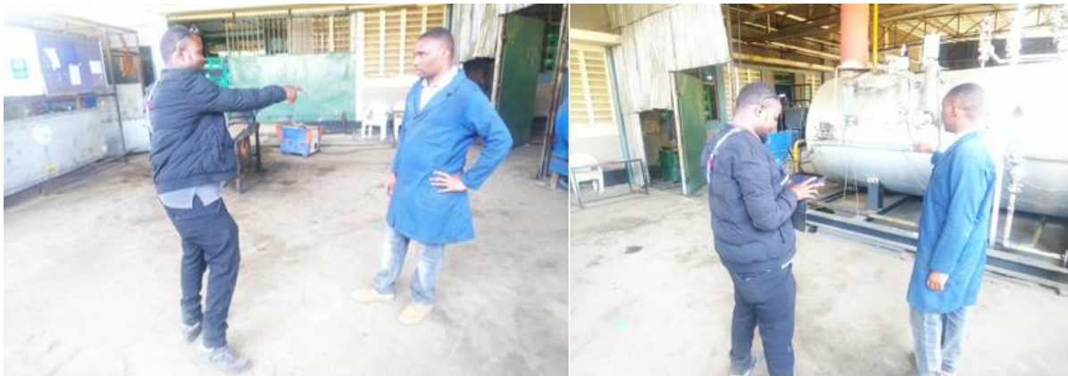
Figure 10: The interview carried out with boiler operator
