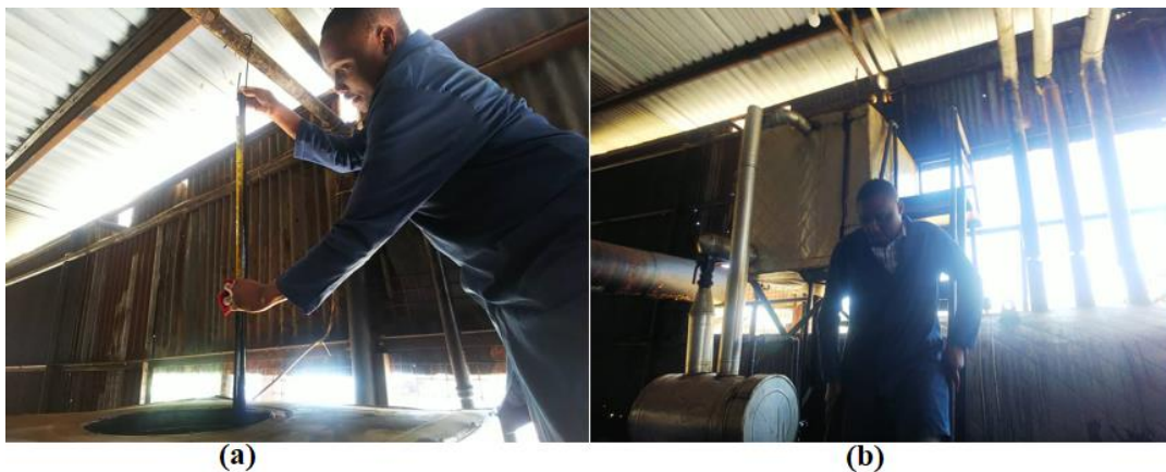
Figure 8: RABEC Fuel monitoring (a) using stick and a manual meter (b) descent of RABEC operator from top of the fuel tank
