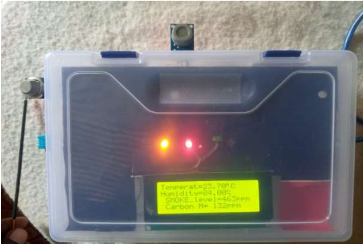
Figure 21: Case of smoke detection by the system
