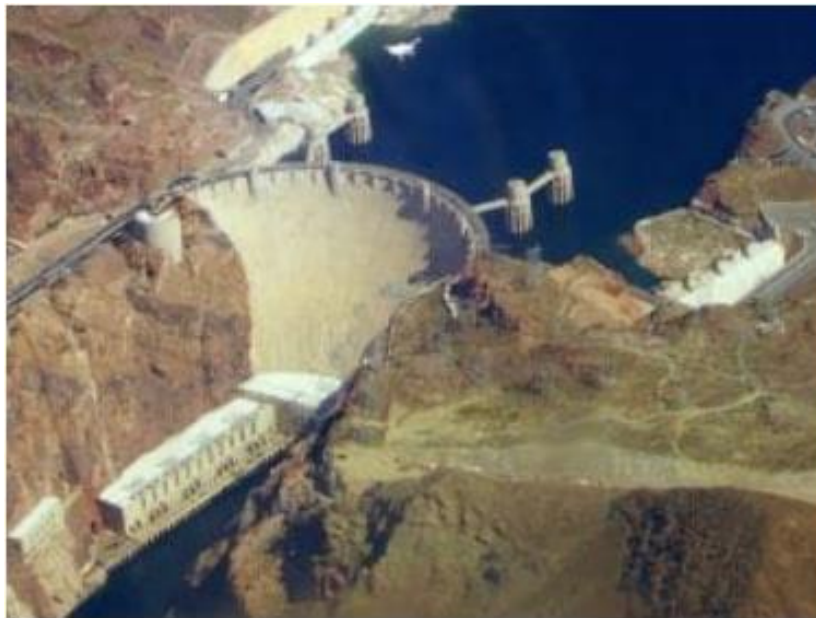
Figure 1: Hoover dam (Tata & Howard, 2022)
