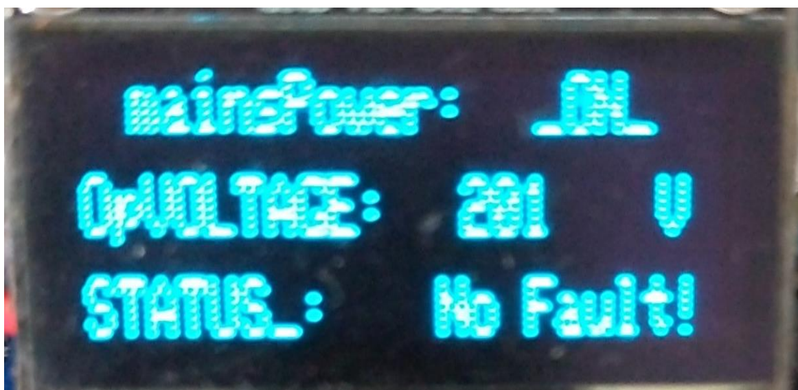
Figure 33: The Main System with UPS being switched on with a Load
