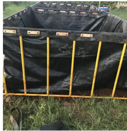
(b) Pond liner attached to the supporting frame
