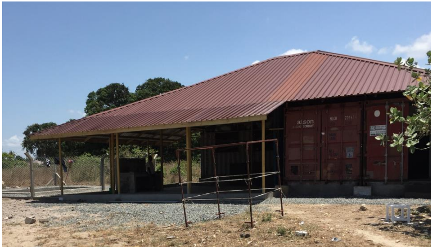
Figure 9: The Bagamoyo IHI LLIN storage facility
