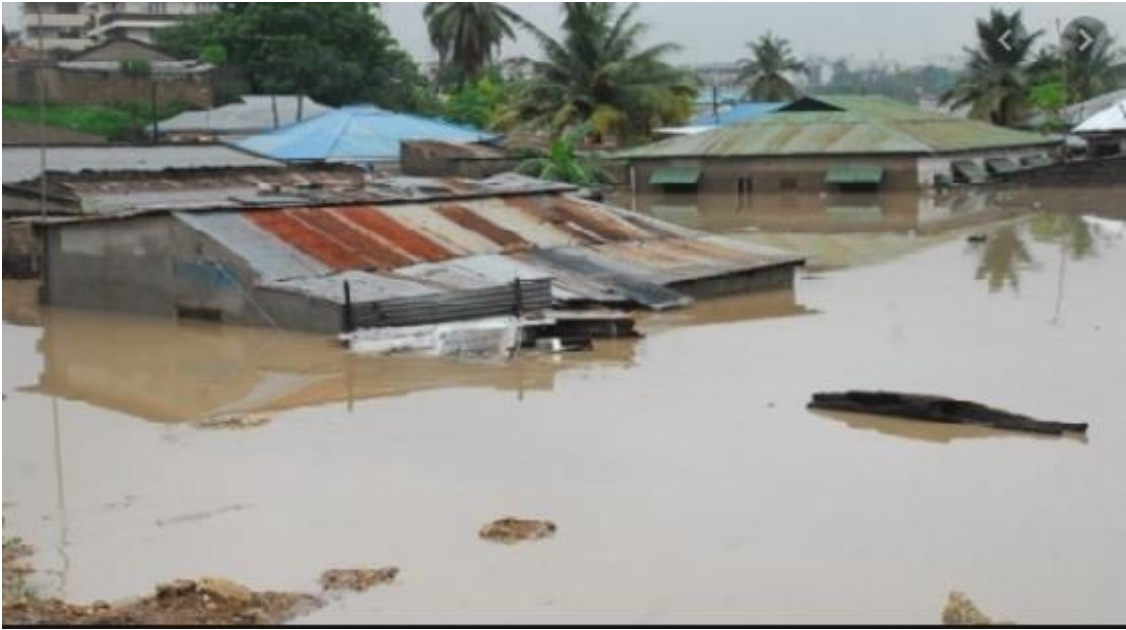
Figure 5: Houses submerged into water (John et al. , 2019)
