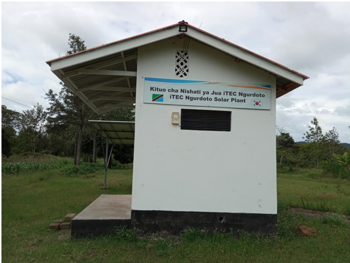
Figure 11: Ngurdoto solar mini-grid centre
