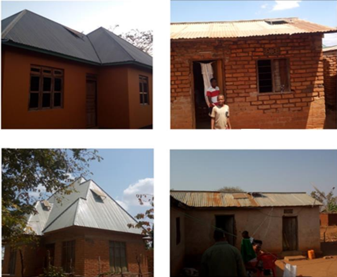
Figure 2: Different roof pitches with dissimilar mounted SPVP on structures in same geographical area
