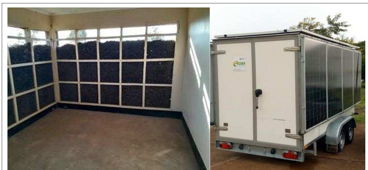
Figure 1: A charcoal cooling room (left) and a walk-in, mobile, solar-powered cold storage unit (right) for storing fresh vegetables
