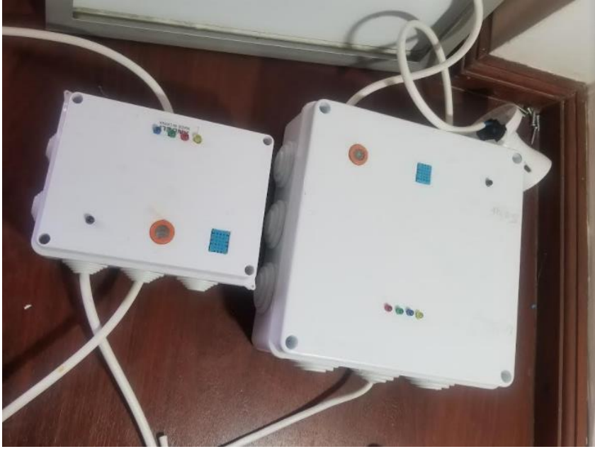
Figure 25: Final prototype for both towers
